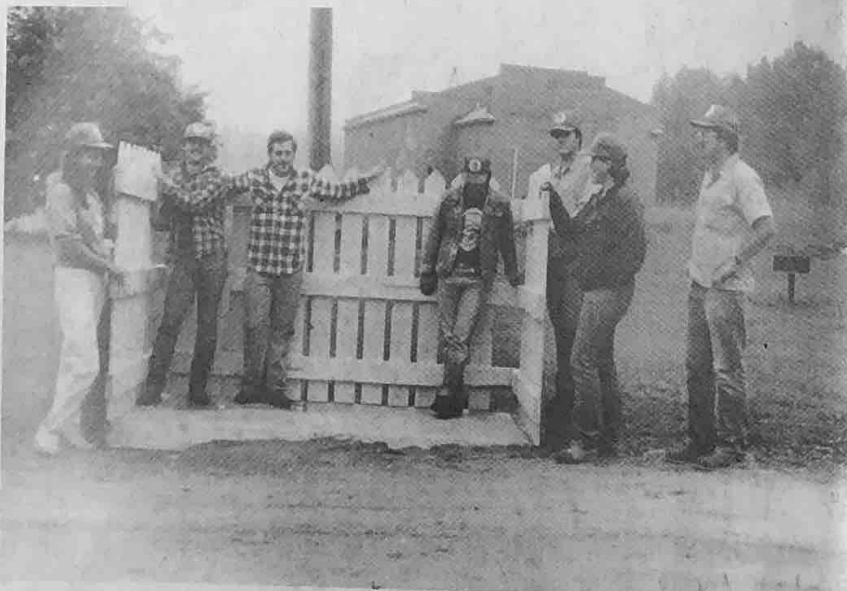
Red Cliff WCC crew are busy erecting pads and vanity fences for a containerized garbage disposal system on the Red Cliff Reservation.
