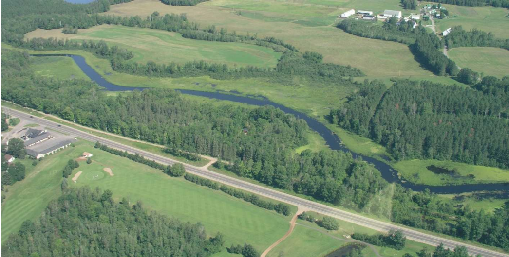
Figure 91. Rat River, North of HWY 8/32, Forest County, 2006.
